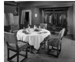
1 North Room, The Jan Martense Schenck House, Brooklyn . Built circa 1675. 50.192, Gift of the Atlantic Gulf and Pacific Company
